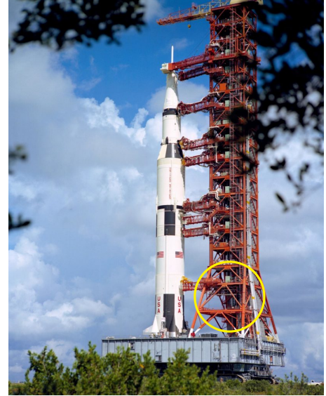
Figure 1: The truss section to be analyzed, and the corresponding part of the launch umbilical tower circled on the Apollo 17 stack (Photo: NASA).
